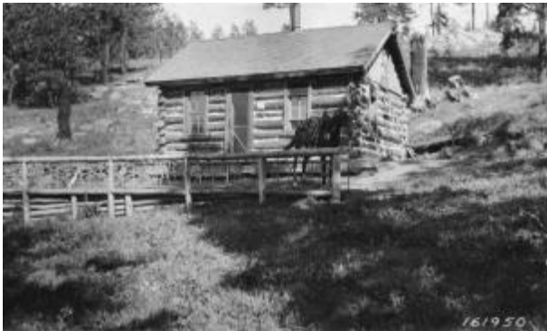
1922 Bear Creek Ranger Station
