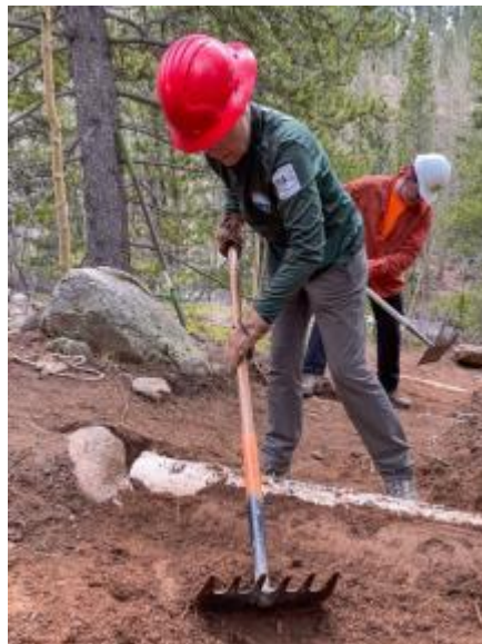
Finishing a water bar Annie
