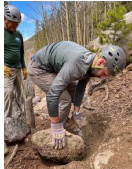
Positioning a stone step L - R: Brian & Wyatt
