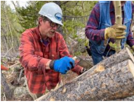
Removing bark with a draw knife Greg
