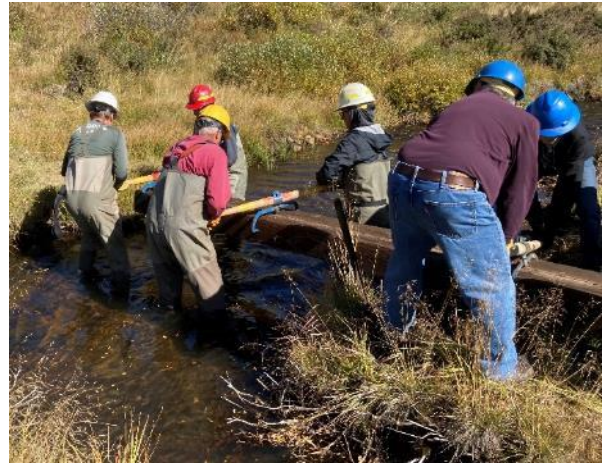
Sliding the bridge into place
